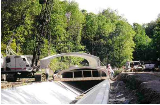
Figure 4.1 – CSO Facility Under Construction (RVA Photo)
